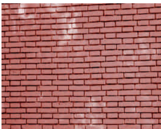
(a) Brick wall
